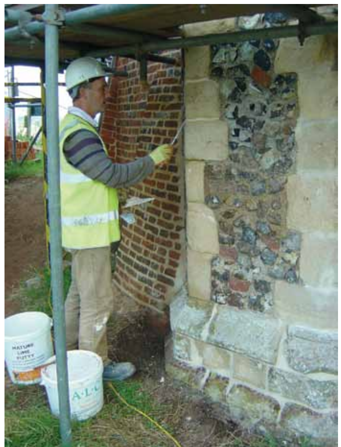
Most of the stonework in the gatehouse was in good order and the joints were just raked out and filled with fresh lime mortar.
