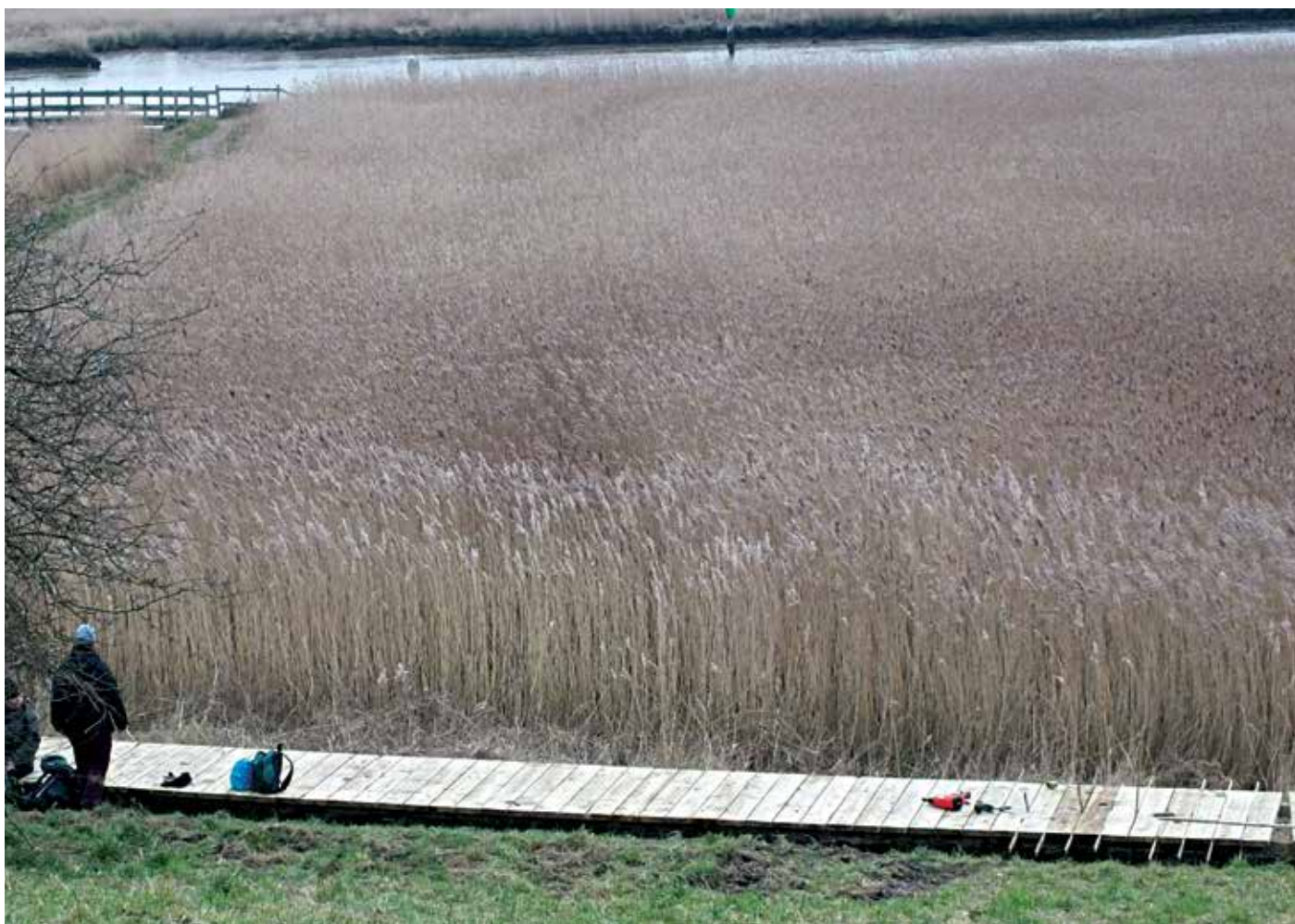
Fig 9: Burgh Castle. The new boardwalk being installed. Photo: Su Waldron
