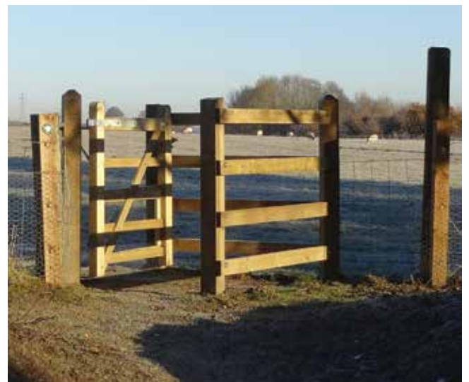
Fig 8: Caistor. New kissing gate
