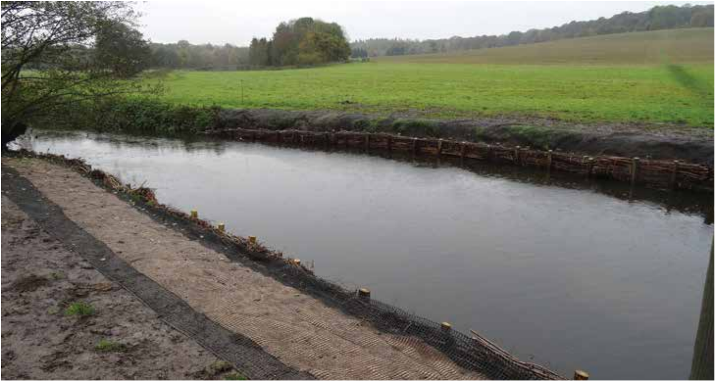
Fig 7: Caistor. River bank repairs.
