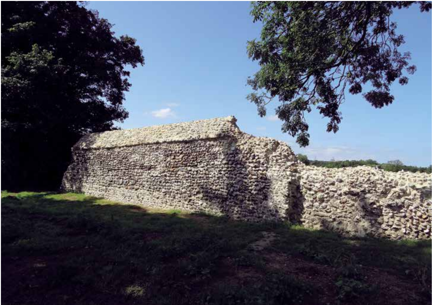
Section of repaired full-height precinct wall at Castle Acre Priory.
