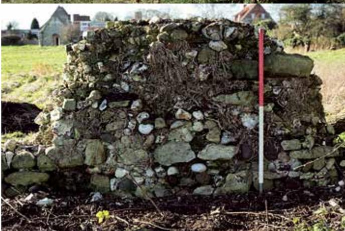
Fig 4: East wall exterior with mixed stones repair. Photo: NPS
